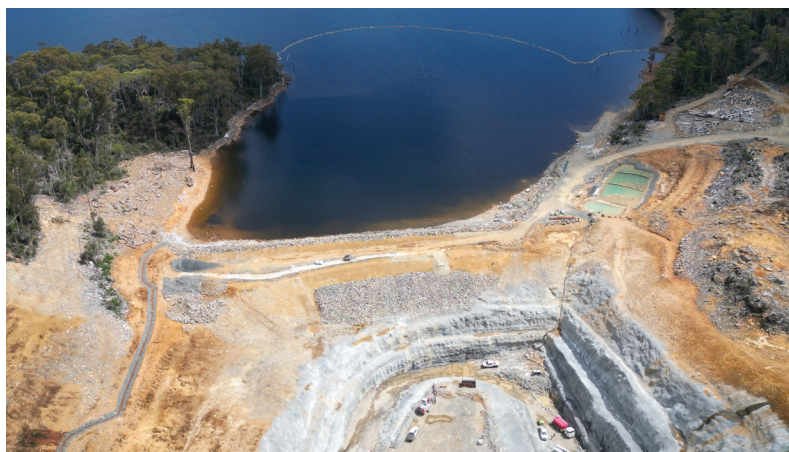
Above: Lake King William intake under construction as part of the upgrade works underway to support a potential redevelopment of the Tarraleah hydropower scheme
